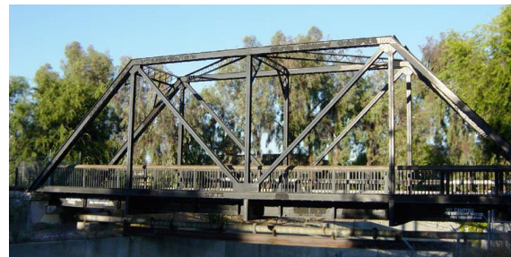
Figure 1- A truss used in the construction of a bridge.
